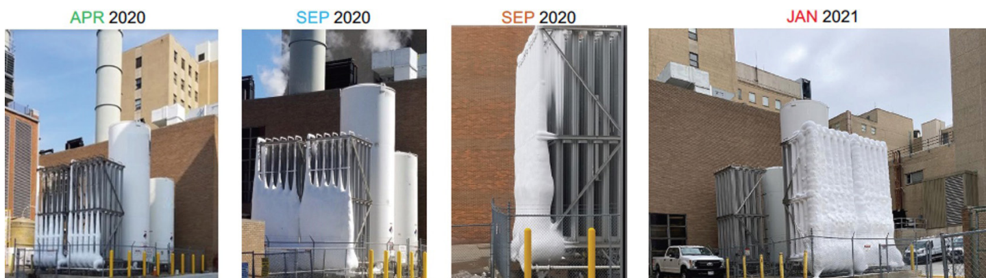
Figure 11. Progressive icing of coils of a hospital-based oxygen system with increased oxygen use during the pandemic. From Chatburn RB, Branson RD. Shortages and vulnerabilities of hospital oxygen systems. Respir Care 2022;67(8):in press.
