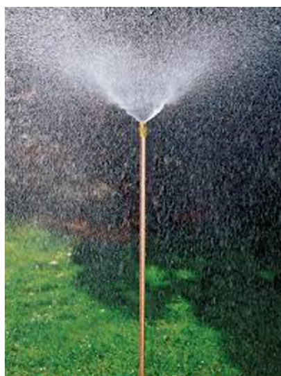
Figure 12. Excessive icing of the piping system leading to the hospital (Top). A mitigation strategy was the use of warm water irrigation sprinklers to intermittently melt ice accumulation.
