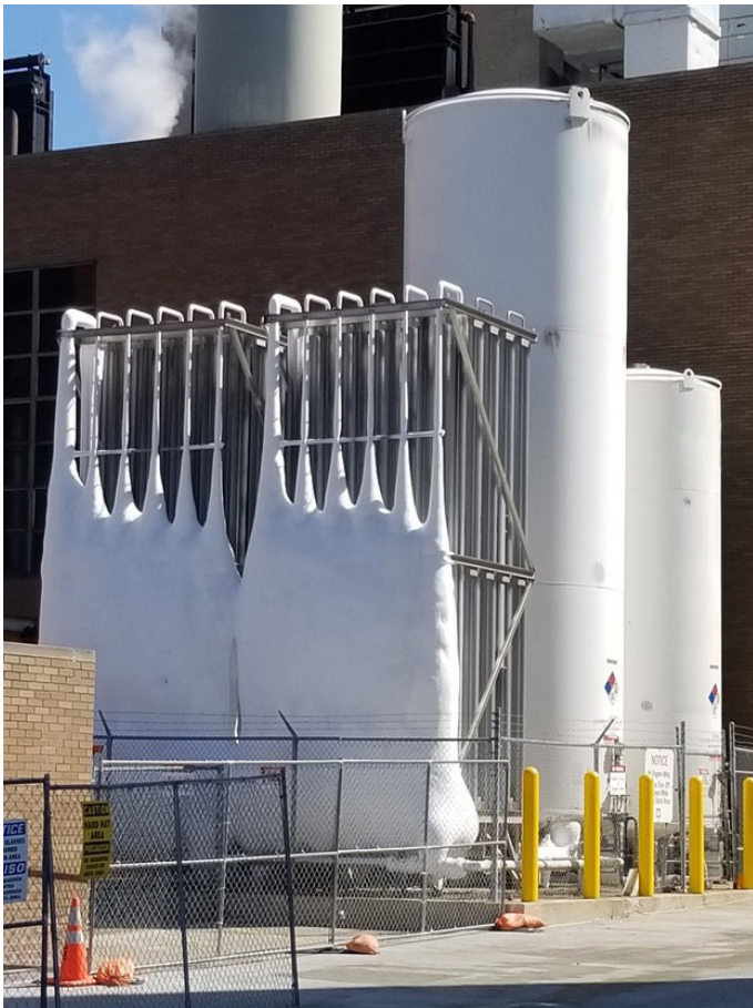
Depiction of a strained liquid oxygen system.
